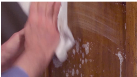
Clean with degreaser / rinse with water
